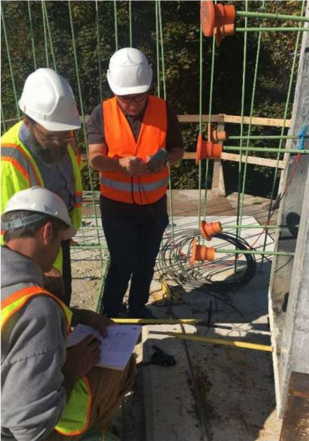
The main advantage of EIT systems is the ability to non-destructively monitor tendon encapsulation over time. In the photo above, initial construction reading is collected.
